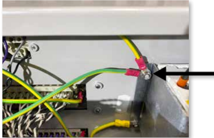
Figure 3-2 Ground connection of the Me controller
