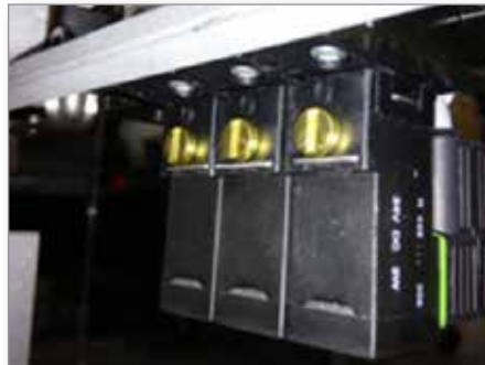
Figure 11-4 Manual override switch
