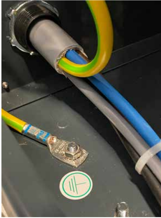
Figure 3-2 Example of a ground connection
