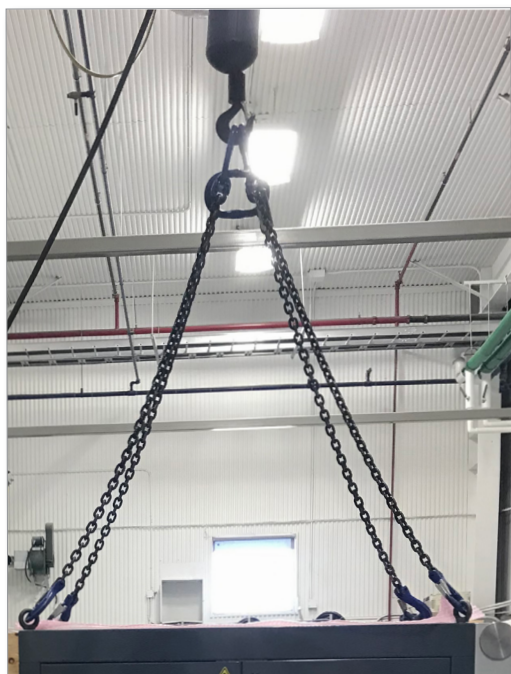
Figure 3-11 Attach slings to all four eyebolts
